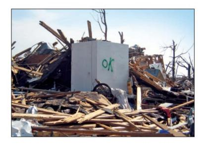
An above-ground residential safe room that was in the garage of a home hit by an EF5 tornado in Joplin, Missouri (2011). This saferoom was built to meet FEMA guidance, which offers near-absolute life-safety protection, so the occupants were unharmed even though their house was destroyed.
