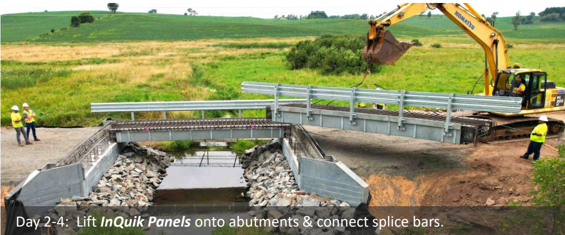
InQuik modular components (abutments & panels) are pre-fabricated offsite.
