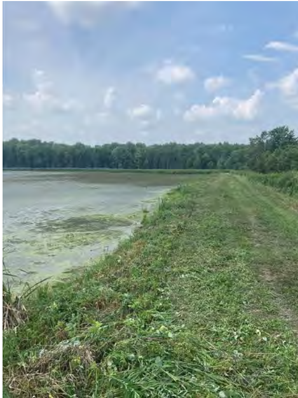
Picture 1. Bern dike after mowing and brush cutting.
