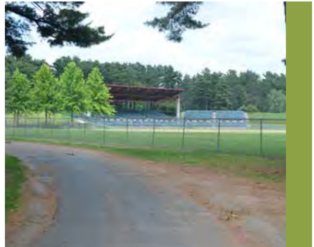
Feature 22: Existing Grandstand
