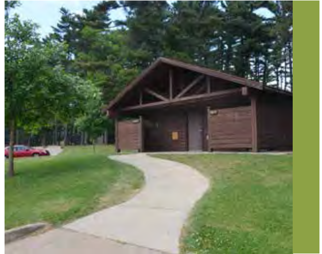
Existing Restrooms north of Grandstand (to be maintained)
