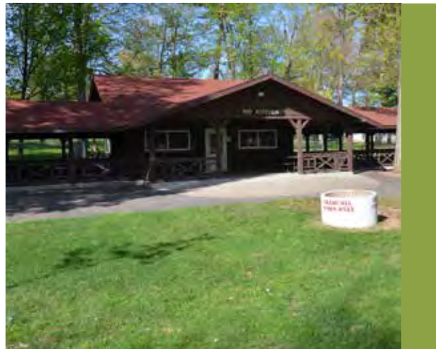
Feature 10: Existing Big Kitchen Building
