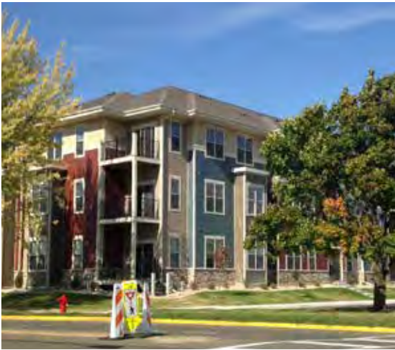
Feature 35: Residential Redevelopment - Apartments
