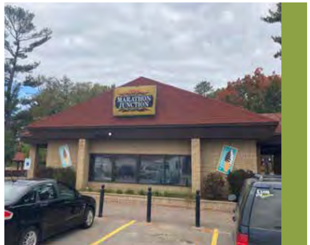
Feature 6: Existing Marathon Junction Building
