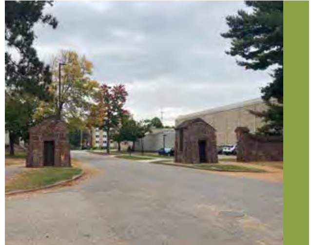
Feature 13: Existing East Pedestrian Entrance
