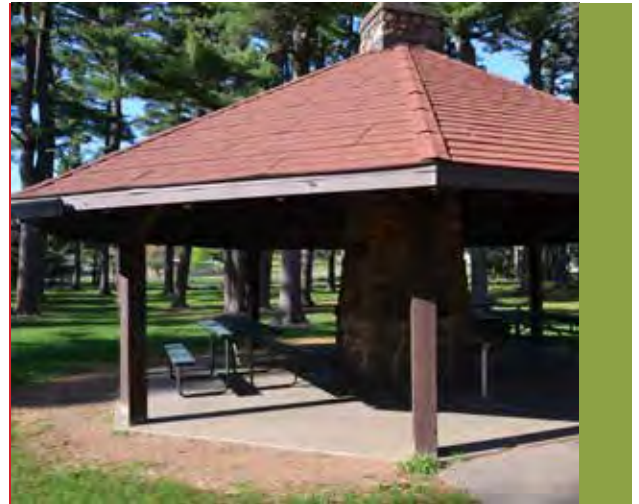
Existing Shelter east of Campground (to be maintained)
