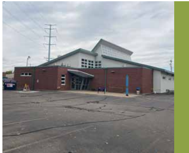
Feature 18: Existing Arts Building
