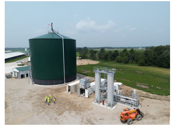
Red Leaf RNG Project at Maple Row Dairy (Operational)
