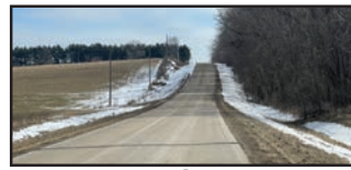
⑤ Steep slopes, narrow R.O.W., and adjacent wetlands may impact off-road trail space.
