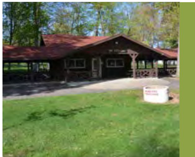
Feature 10: Existing Big Kitchen Building
