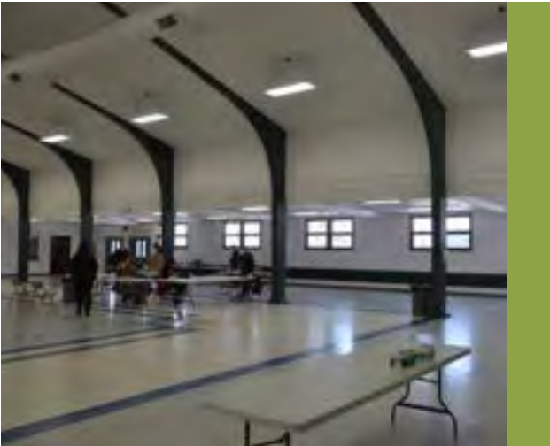
Feature 14: Existing East Gate Hall Interior
