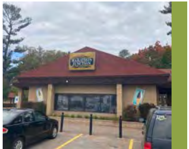
Feature 6: Existing Marathon Junction Building
