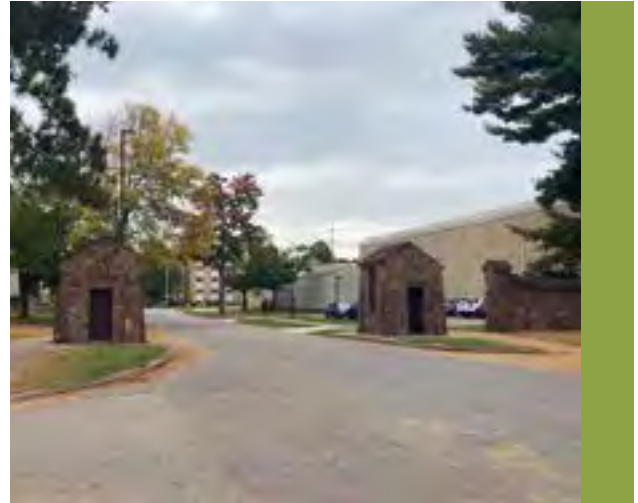
Feature 13: Existing East Pedestrian Entrance
