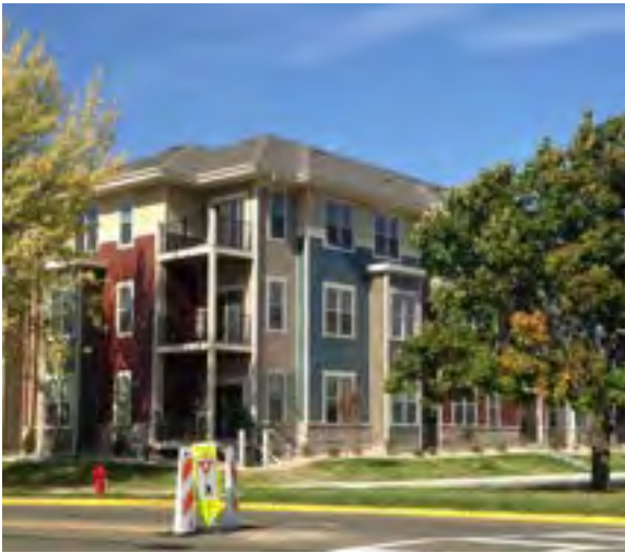
Feature 35: Residential Redevelopment - Apartments
