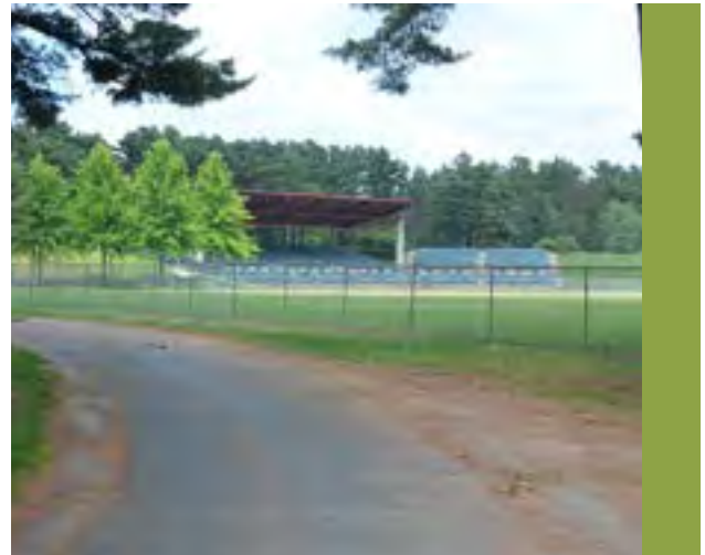
Feature 22: Existing Grandstand
