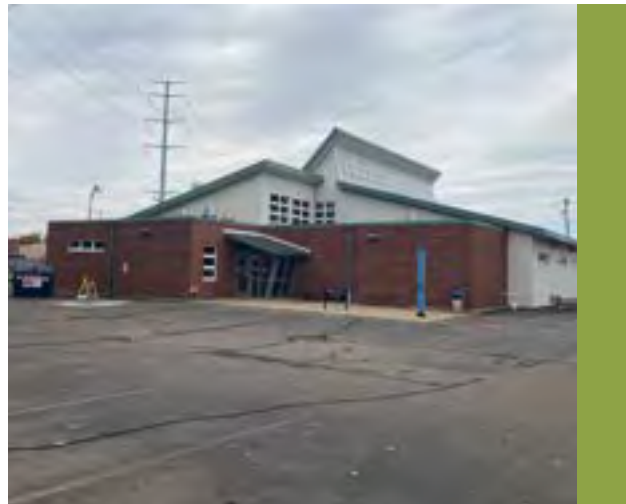
Feature 18: Existing Arts Building
