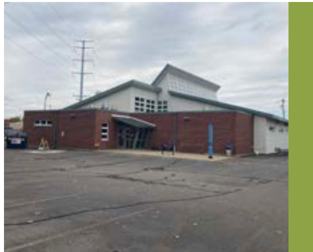
Feature 18: Existing Arts Building
