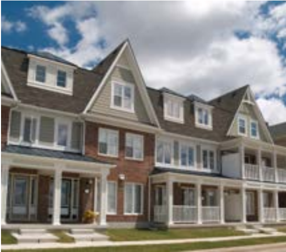
Features 32/34: Residential Redevelopment - Townhomes
