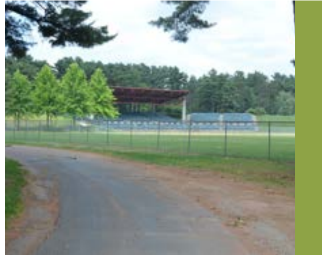
Feature 22: Existing Grandstand
