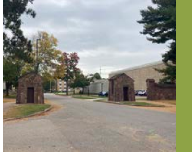
Feature 13: Existing East Pedestrian Entrance
