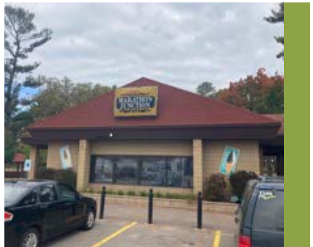
Feature 6: Existing Marathon Junction Building
