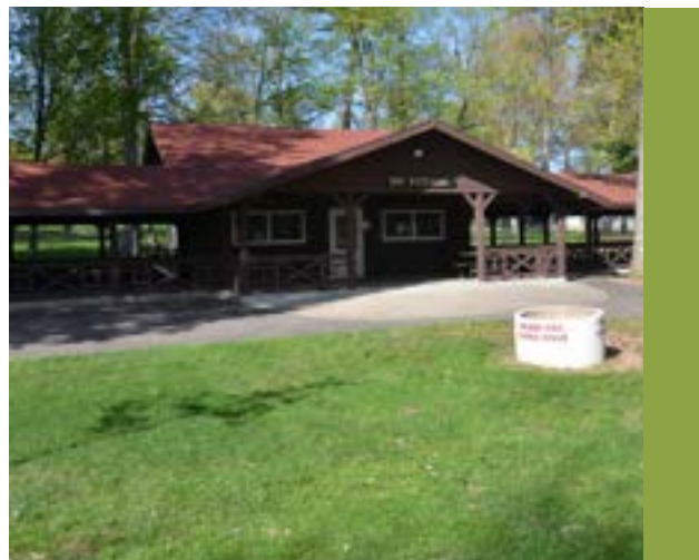
Feature 10: Existing Big Kitchen Building
