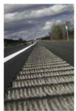
Rumble strips are an engineering treatment designed to alert drivers of a lane departure through vibration and noise created when a vehicle's tires contact the rumble strip. Shoulder and centerline rumble strips on rural two-lane roads are especially helpful during bad weather such as rain, snow or fog when visibility of the edge line or centerline is reduced. Rumble strips also help to
