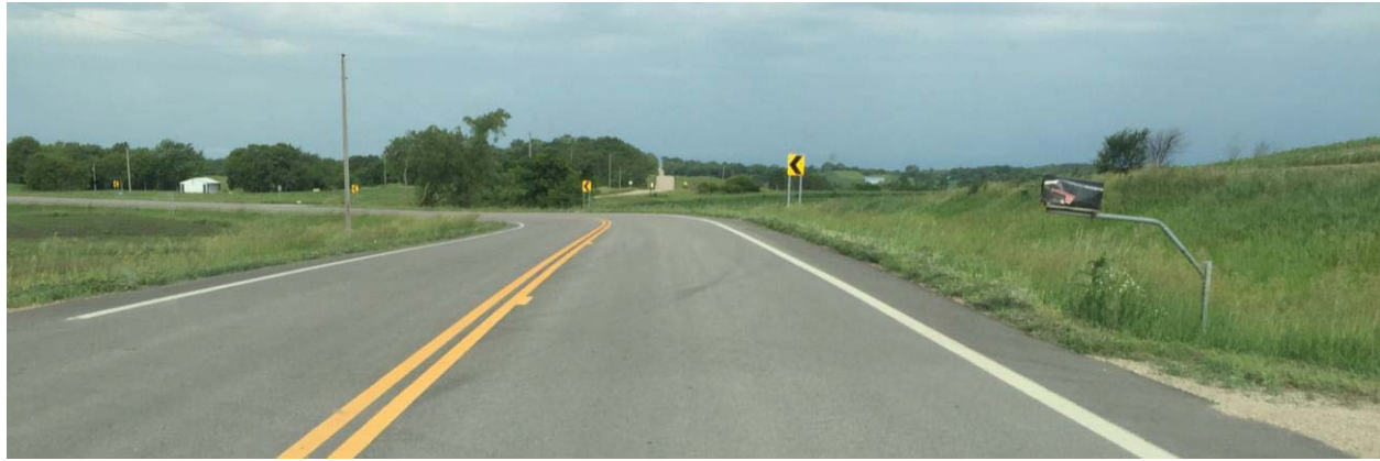
Figure 11. Visual Trap on a Curve
