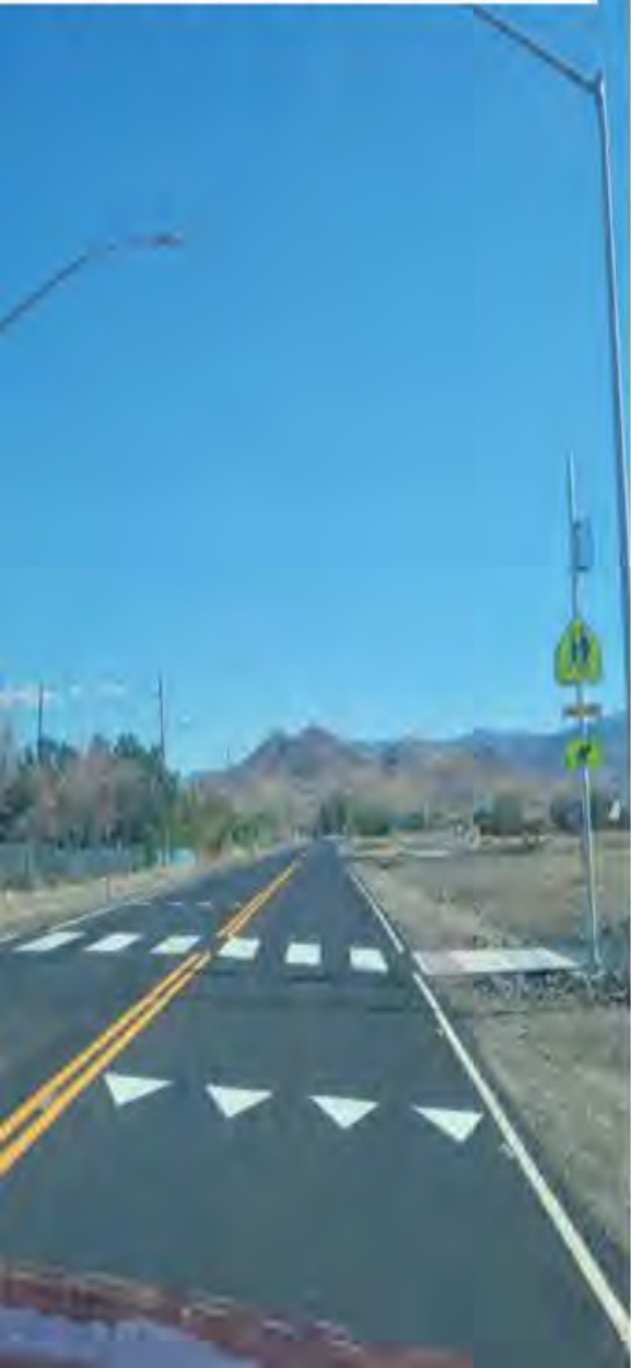
Figure 10. Crosswalk visibility enhancements include advance yield markings, high visibility crosswalk markings, lighting, and a rectangular rapid flashing beacon. Source: FHWA
