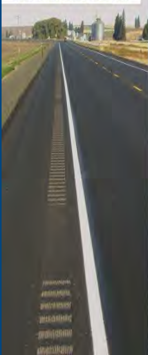
Figure 4. Shoulder rumble strips. Source: FHWA
