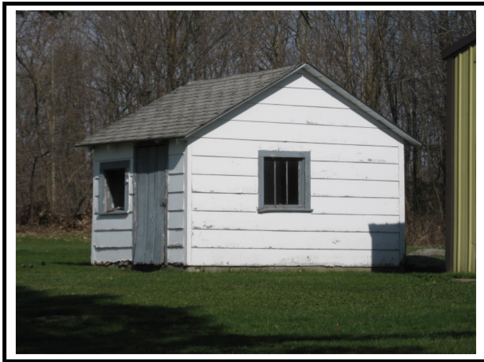
11. Front view of shed.
