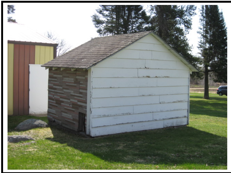
12. Rear view of shed.
