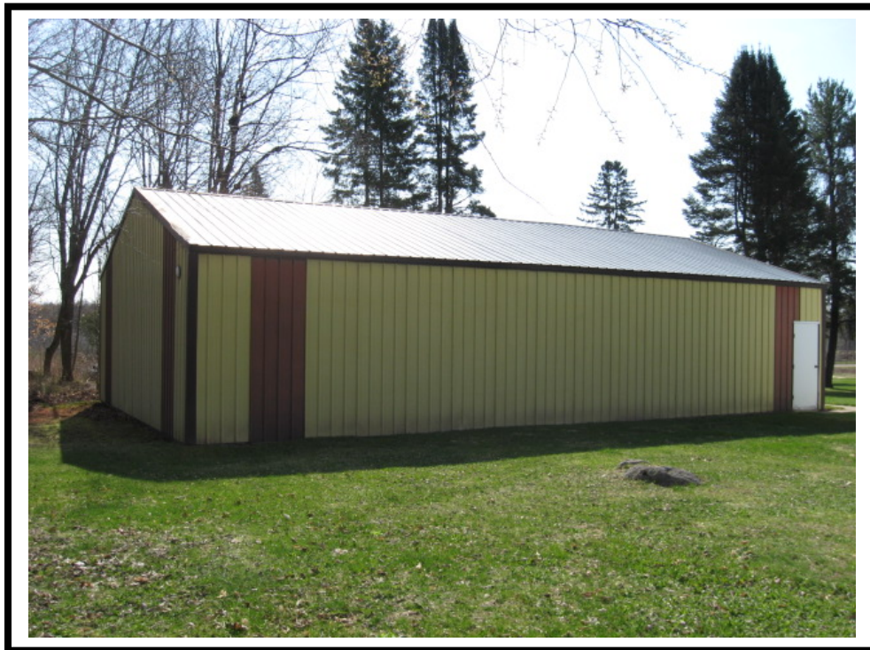
14. Rear view of pole building.
