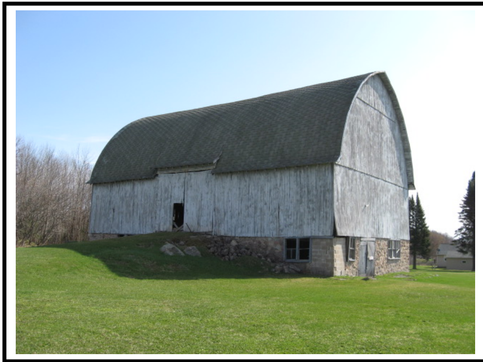
16. Rear view of barn.
