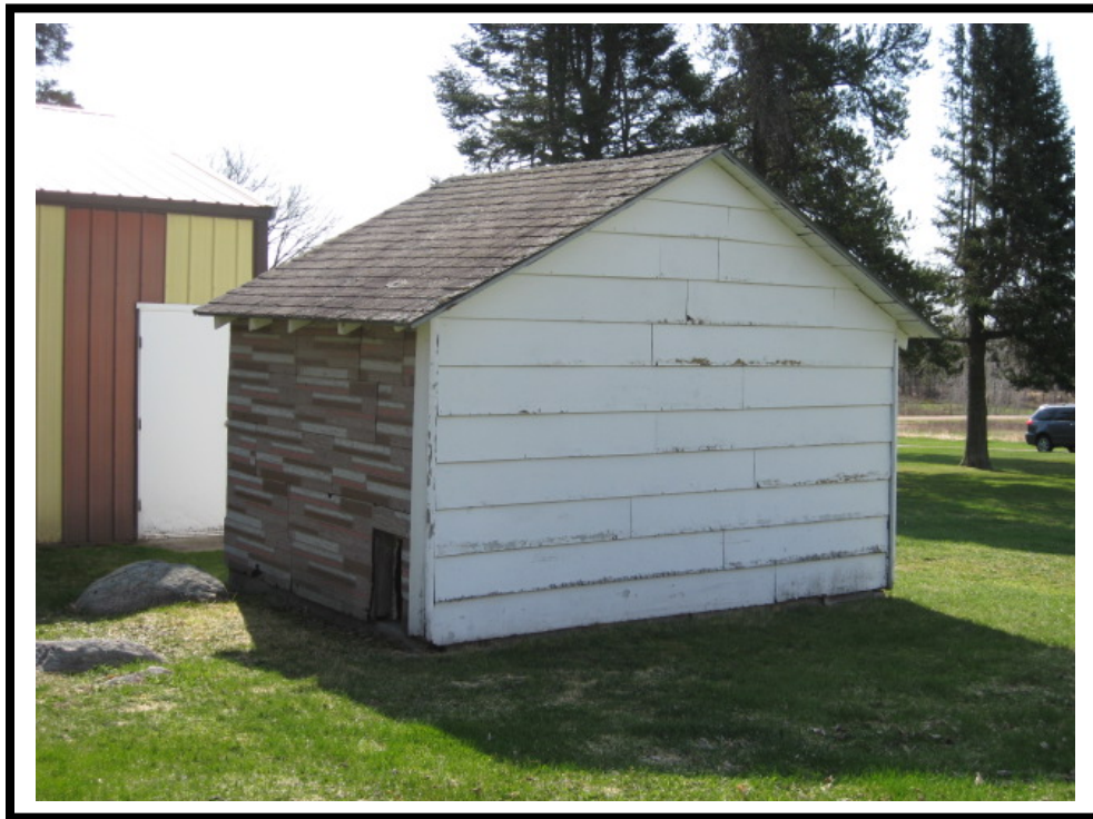
12. Rear view of shed.
