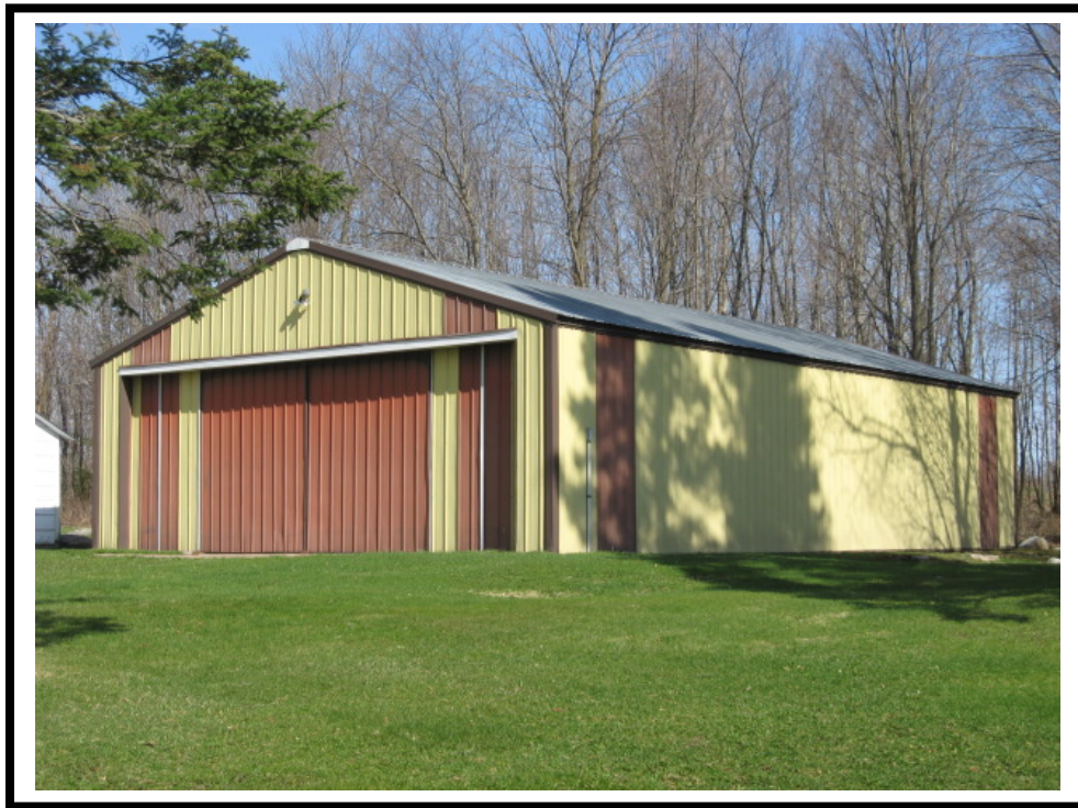
13. Front view of pole building.
