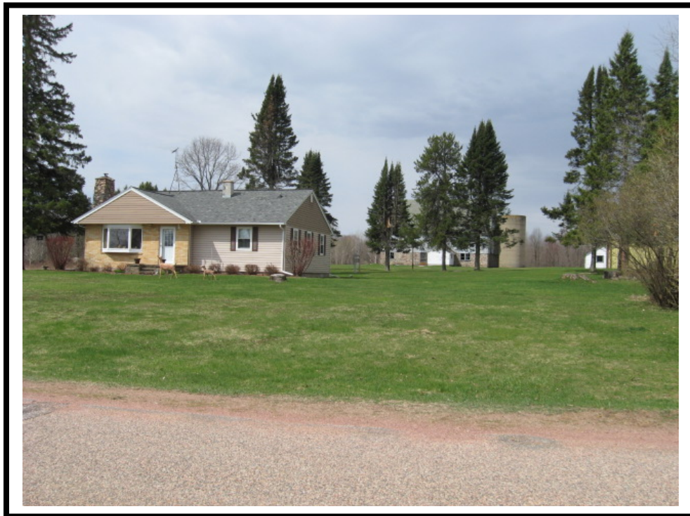
28. View looking west from Duncan Road at buildings.
