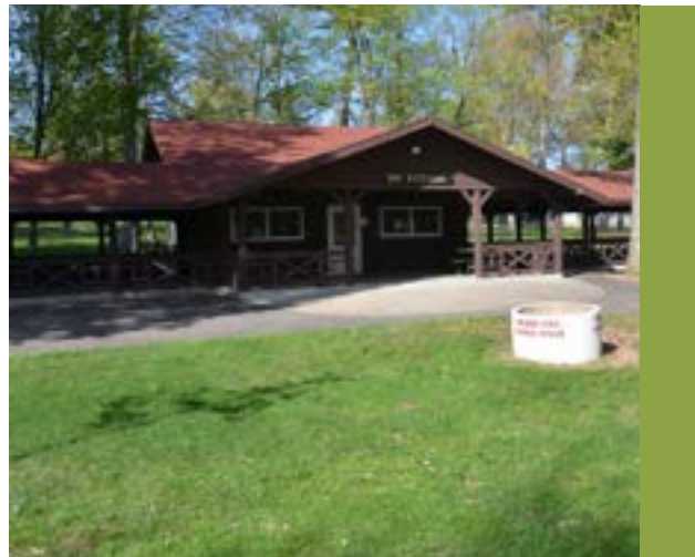
Feature 10: Existing Big Kitchen Building
