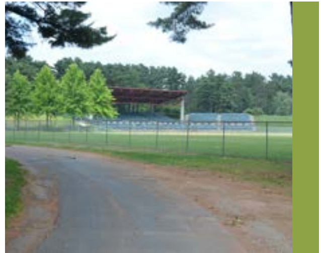
Feature 22: Existing Grandstand
