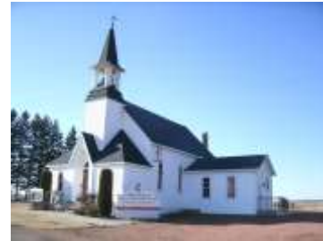
Rib Falls United Methodist Church
