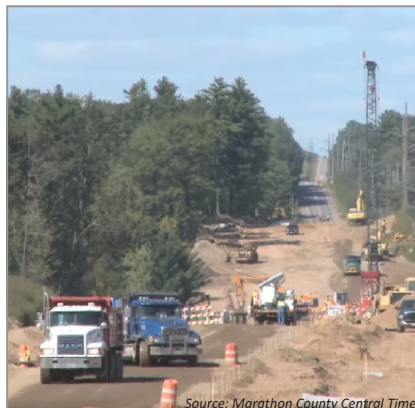
Road construction and repair.
