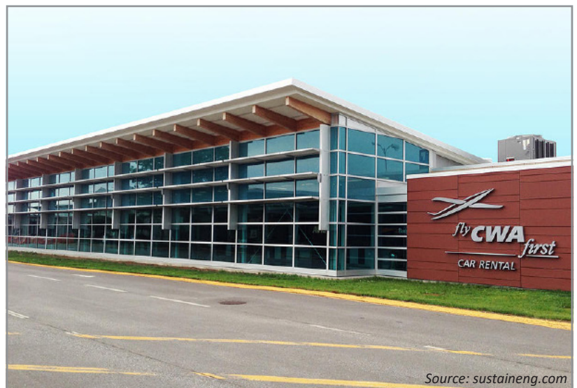
Central Wisconsin Airport.
