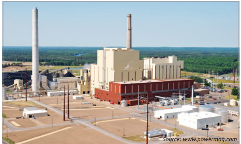
The Weston 4 power plant.
