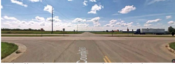
Site of Possible Interchange or overpass at CTH S and STH 29 (southward view from Town of Rib Falls along STH S). Source: Google Street View, 2017
