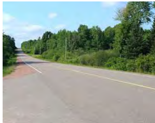
County Highway WW
