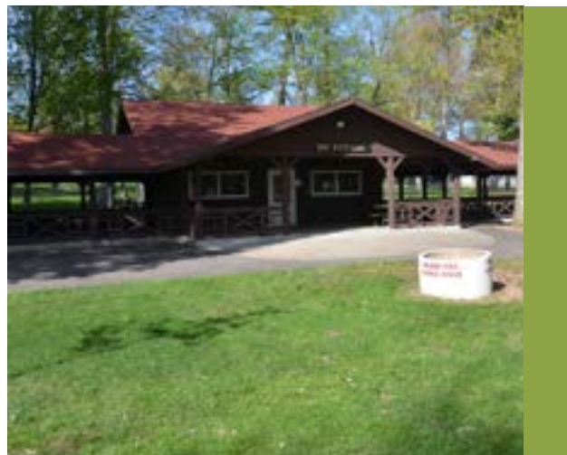
Feature 10: Existing Big Kitchen Building
