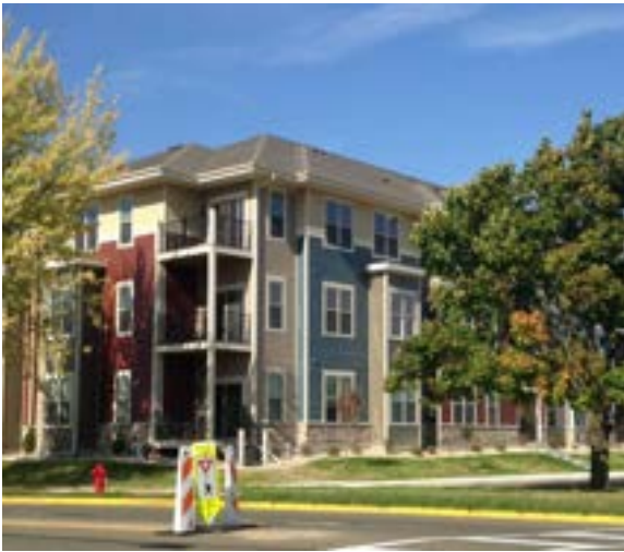
Feature 35: Residential Redevelopment - Apartments
