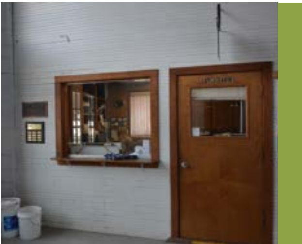
Feature 15: Interior (Fair Office) of Existing Exhibition Building
