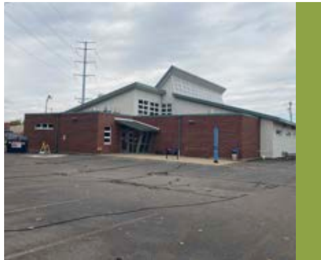
Feature 18: Existing Arts Building
