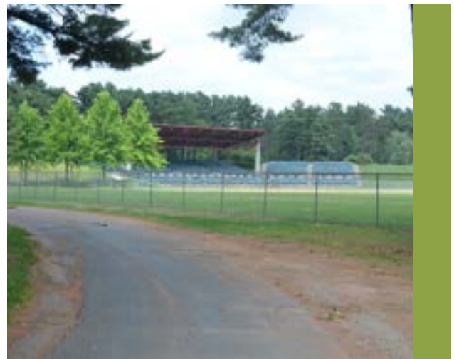
Feature 22: Existing Grandstand
