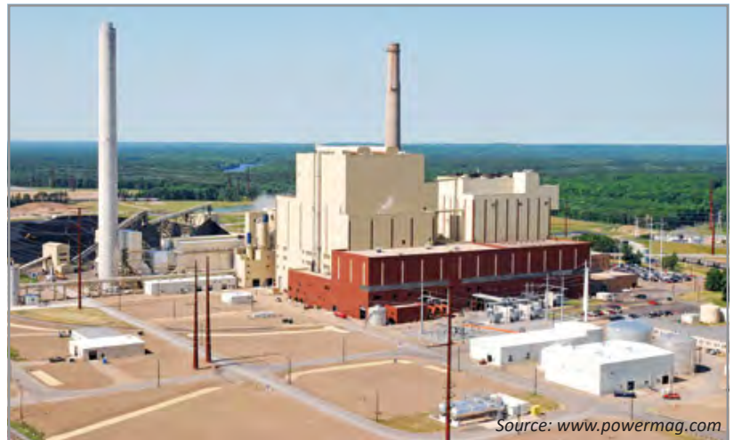
The Weston 4 power plant.
