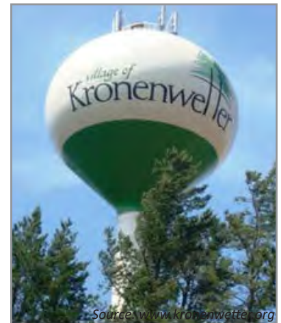
Source: www.kronenwetter.org Water towers are an element of a public water utility's infrastructure.
