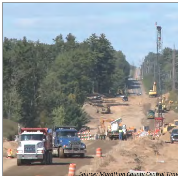
Road construction and repair.
