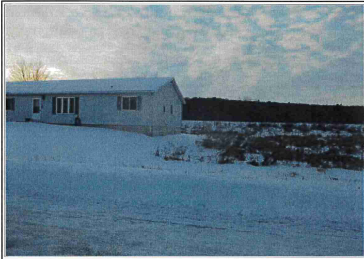
REAR OF SUBJECT PROPERTY
