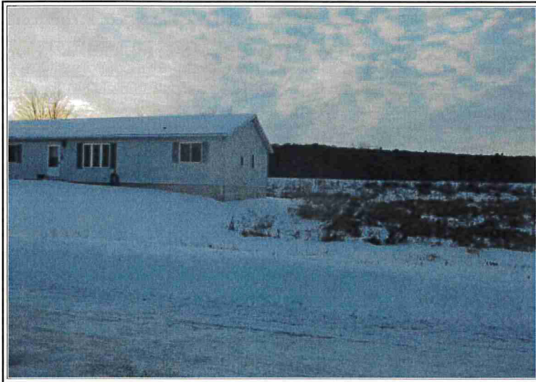
REAR OF SUBJECT PROPERTY
