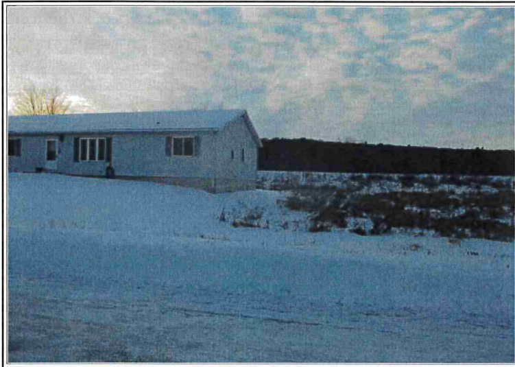
REAR OF SUBJECT PROPERTY
