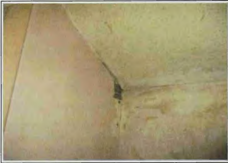
UPPER BEDROOM CEILING
