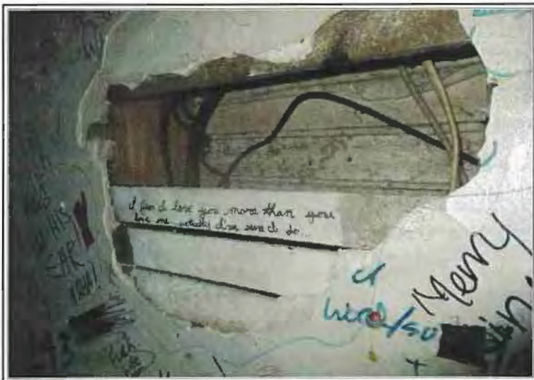
WALL SAME BEDROOM
