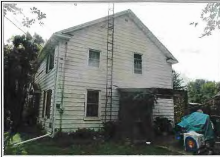
REAR OF SUBJECT PROPERTY
