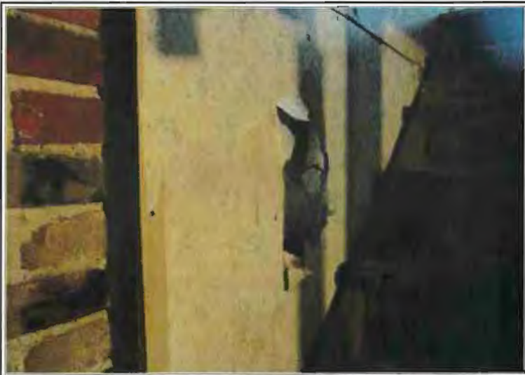
WALL IN BASEMENT STAIRS
