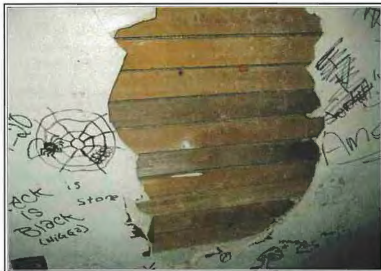
WALL IN BEDROOM
