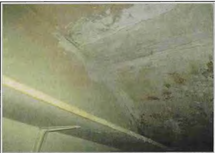
UPPER CLOSET CEILING
