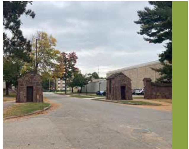
Figure #: Existing West Pedestrian Entrance
