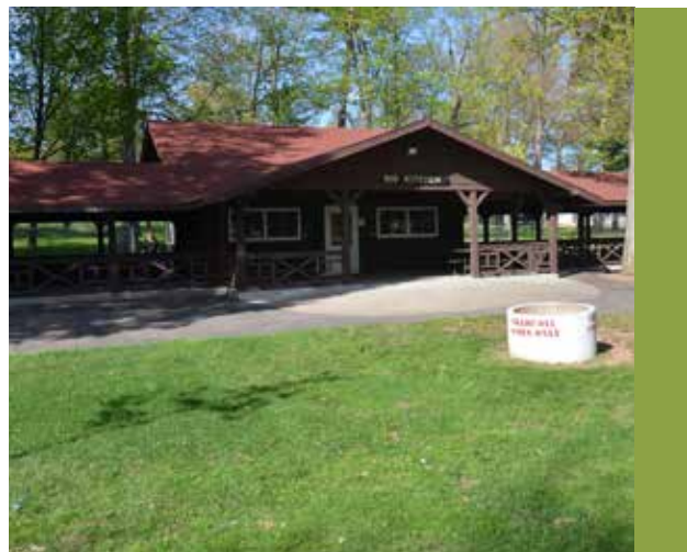
Figure #: Existing Big Kitchen Building
