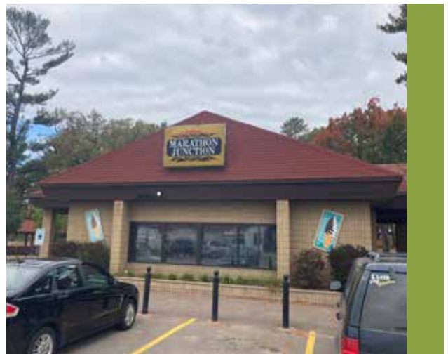
Figure #: Existing Marathon Junction Building
