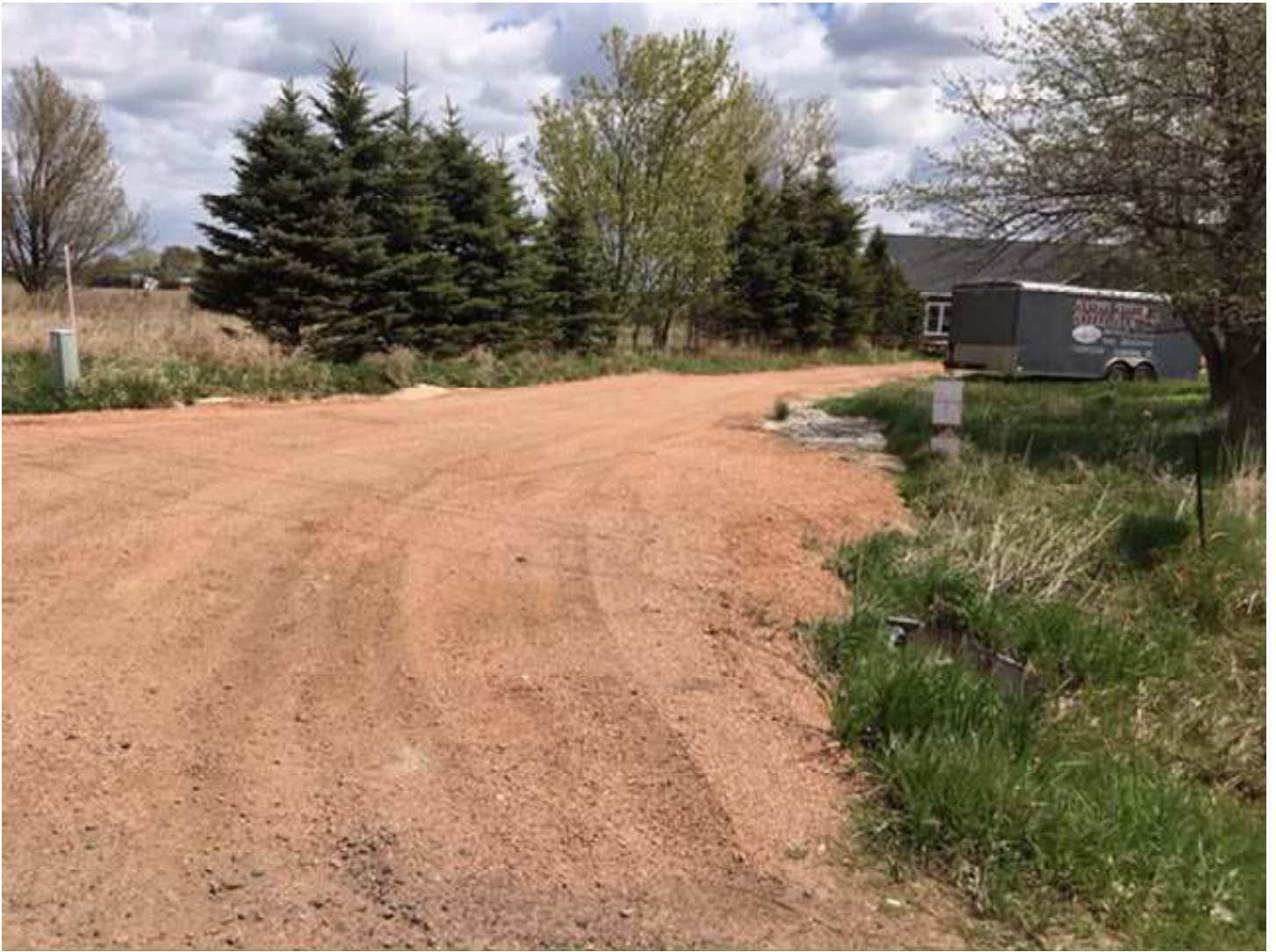
5/6/21 - New Driveway access North of Property.
