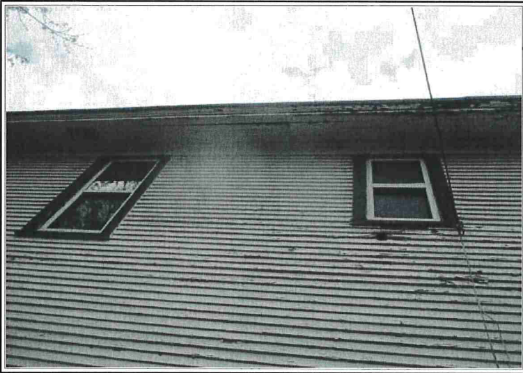
SIDING AND SOFFITS
