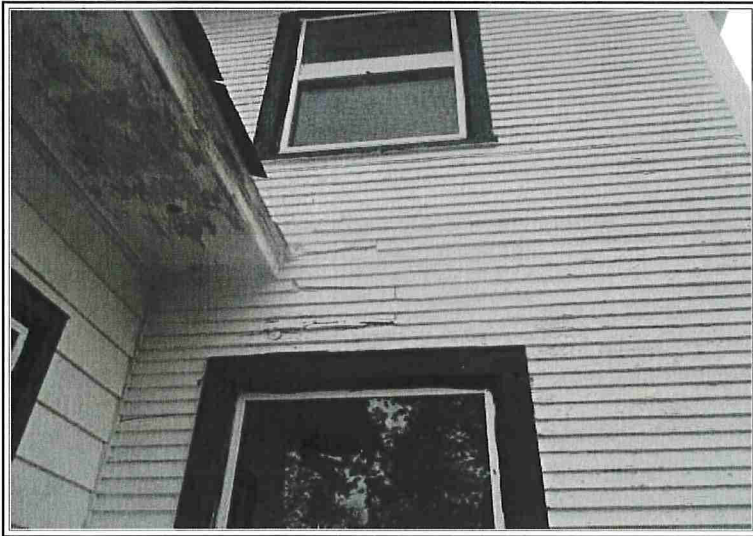
REAR OF SUBJECT PROPERTY
