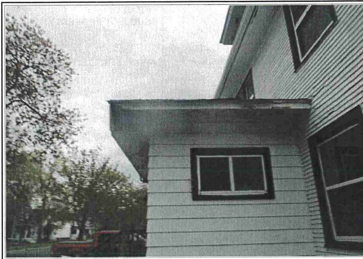
FRONT ADDITION SOFFIT
