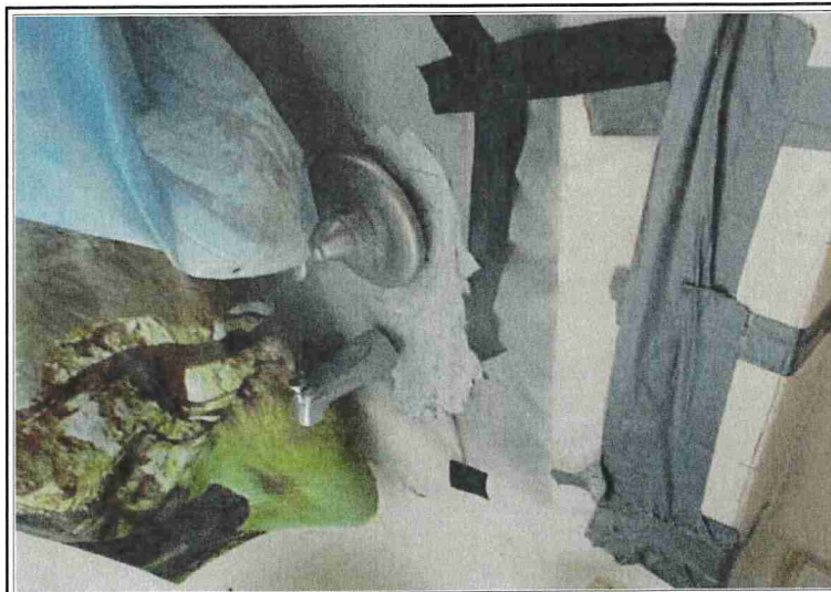
WALL AROUND TUB LOWER
