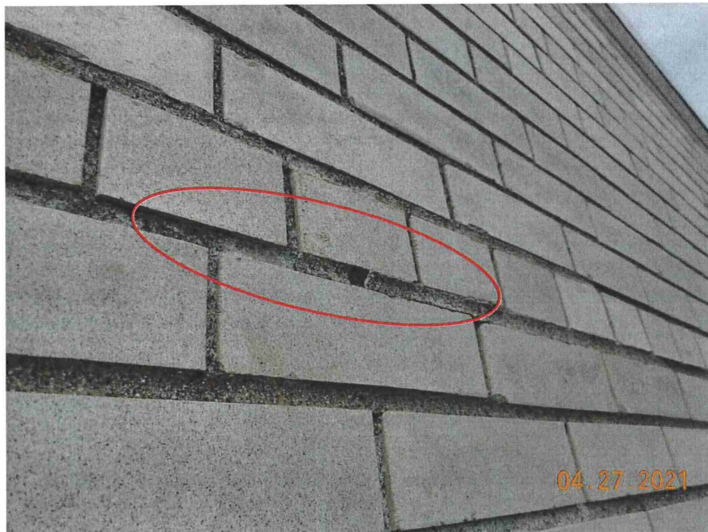
Photo #38: The old tuck point mortar is loose in some areas, but not wide spread.
