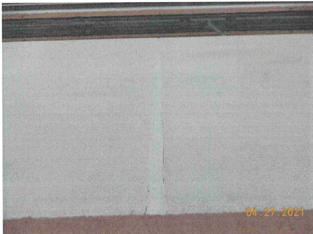
Photo #69: Grind out and replace mortar with silicone sealant.
