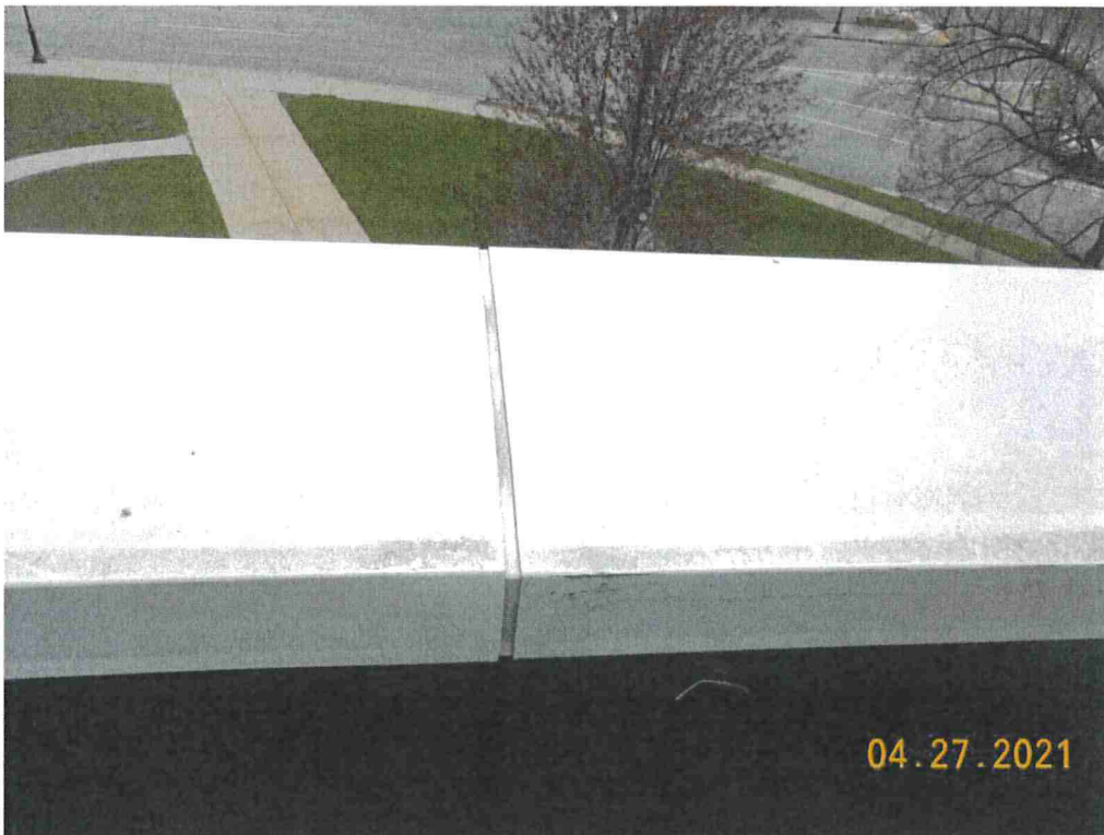
Photo #62: Coping is not typically caulked at the splice joints, only at that southeast corner.
