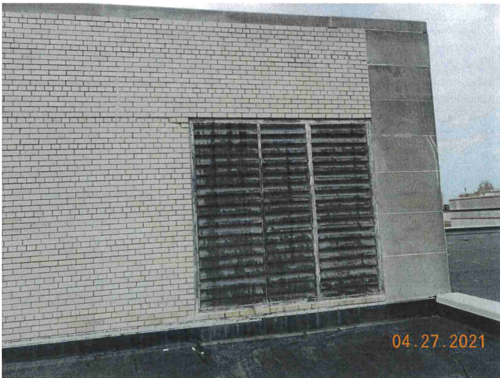
Photo #42: If this louver is not active cover it with composite panel.
