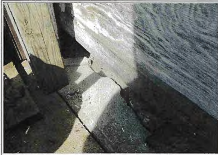
GARAGE DOOR AND FLOOR
