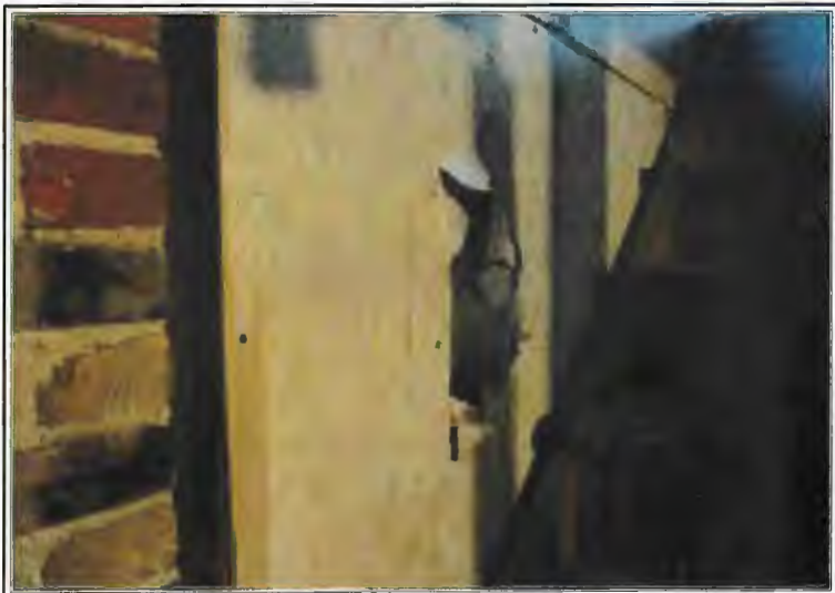
WALL IN BASEMENT STAIRS
