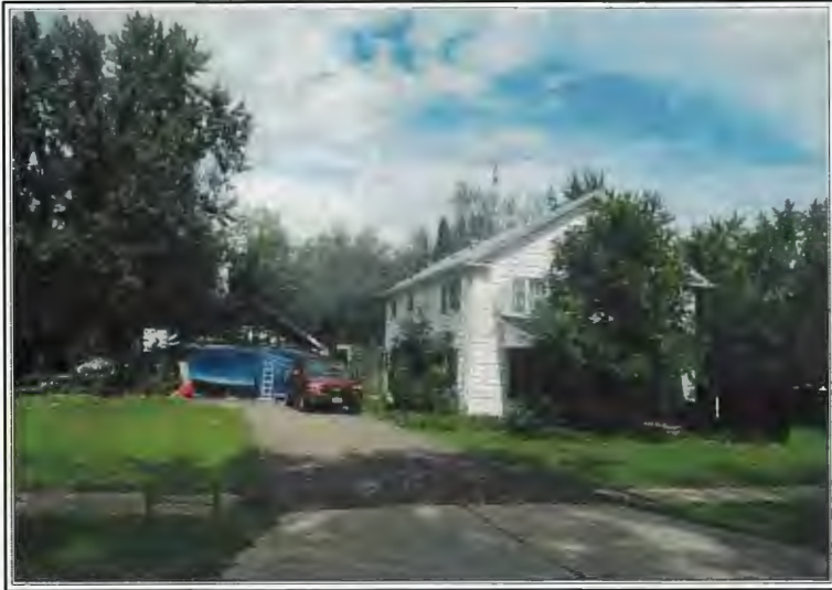
FRONT OF SUBJECT PROPERTY 404 W MAIN ST SPENCER, WI 54479
