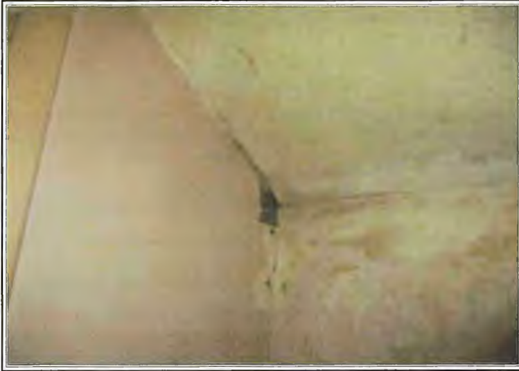
UPPER BEDROOM CEILING
