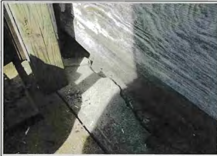
GARAGE DOOR AND FLOOR
