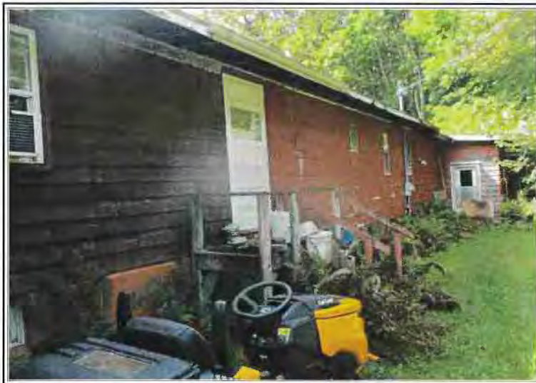
REAR OF SUBJECT PROPERTY
