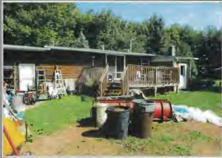
FRONT OF SUBJECT PROPERTY 234495 FIRE STATION RD WAUSAU, WI 54403
