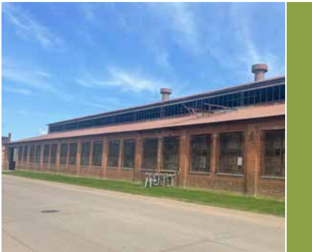
Feature 38: Wausau Iron Works Building (Potential Adaptive Reuse Opportunity)
