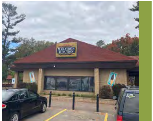
Feature 6: Existing Marathon Junction Building
