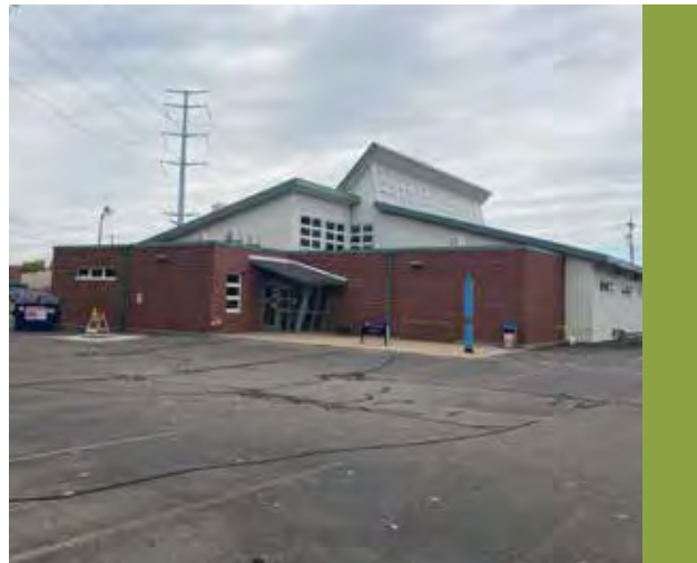
Feature 18: Existing Arts Building
