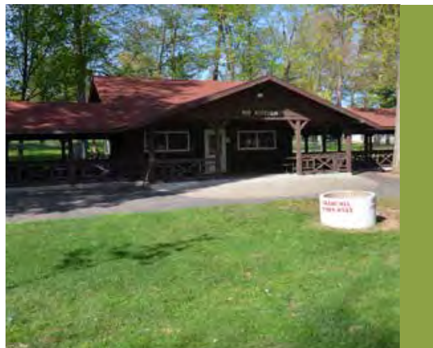
Feature 10: Existing Big Kitchen Building
