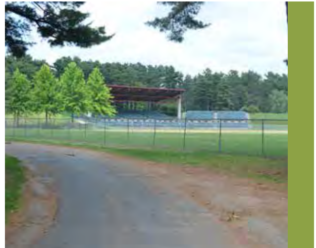
Feature 22: Existing Grandstand
