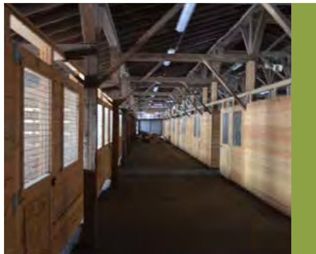
Feature 20: Existing Horse Barn (Interior)
