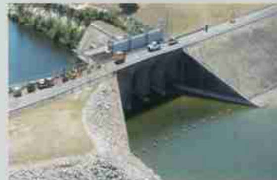
Eagle Mountain Dam and Levee Fort Worth, TX
