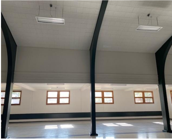
clear story added to mirror the lower level
