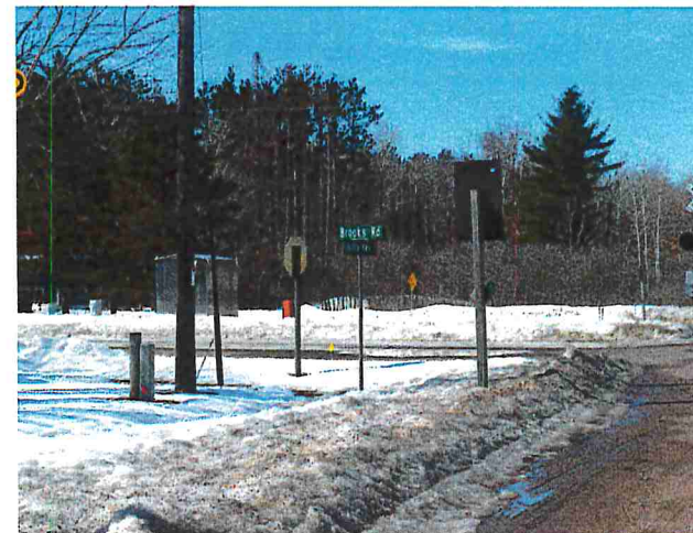
View of Intersection @ RR crossing heading west on City C towards camp
