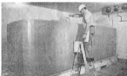
A thick coat of wax to protect Belle was applied by brushes and watering cans.
